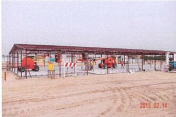
Erection of Steel Structure CFP, MAA Refinery
