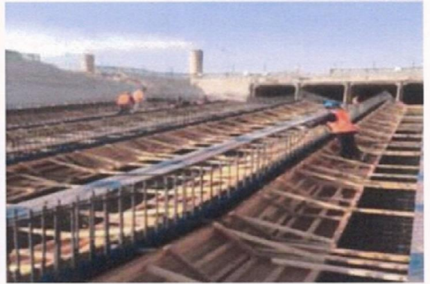
Water Stop Installation IWPP - Az-Zour North
