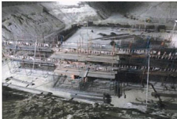
Scaffold Works IWPP - Az-Zour North
