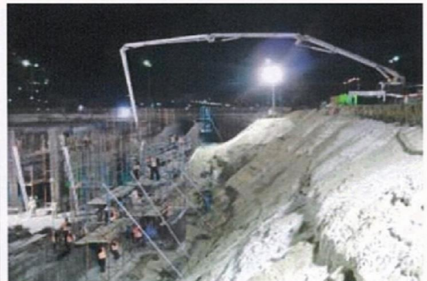
Concrete Placing IWPP - Az-Zour North
