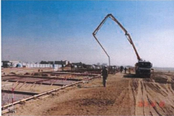
Concrete Foundation Works CFP, MAA Refinery
