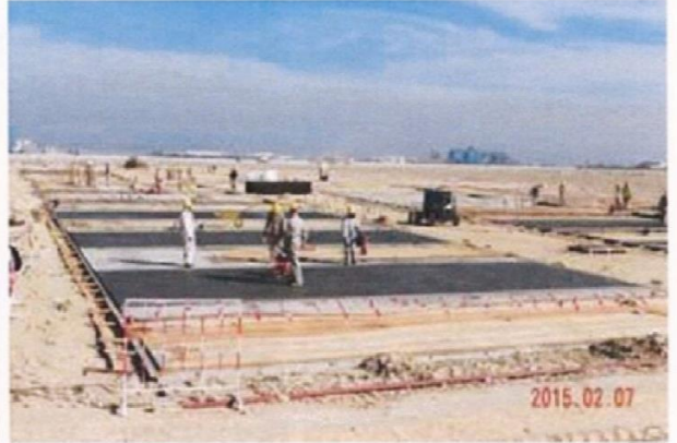
Concrete Foundation Works CFP, MAA Refinery
