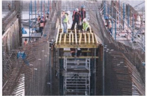
Installation of Top Slab IWPP - Az-Zour North
