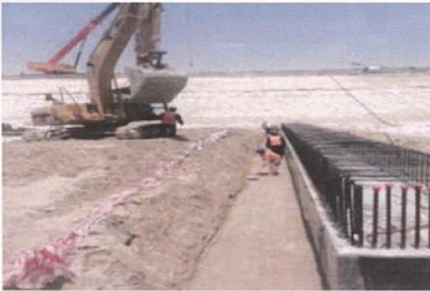
Backfilling Works IWPP - Az-Zour North
