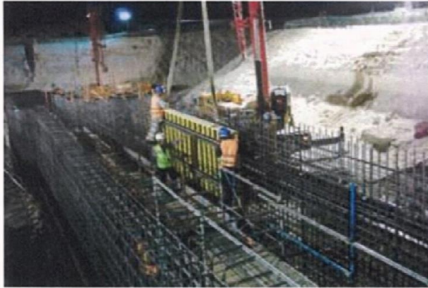
Installation of System Form IWPP - Az-Zour North
