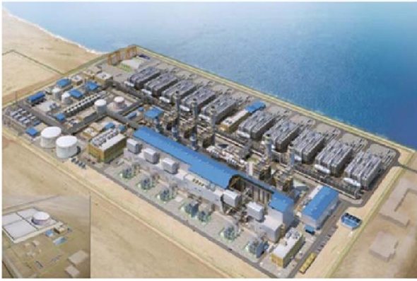
AZ-ZOUR NORTH IWPP PROJECT
