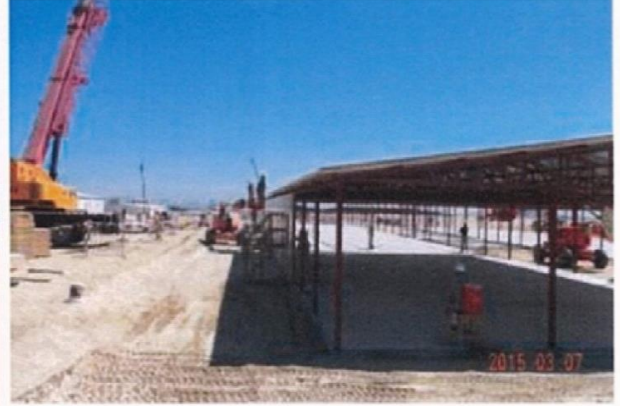
Erection of Roof & Wall Panels CFP, MAA Refinery
