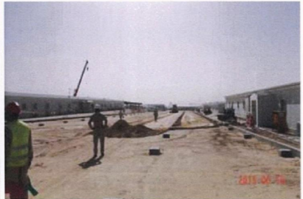
Compaction Work – Road Paving CFP, MAA Refinery
